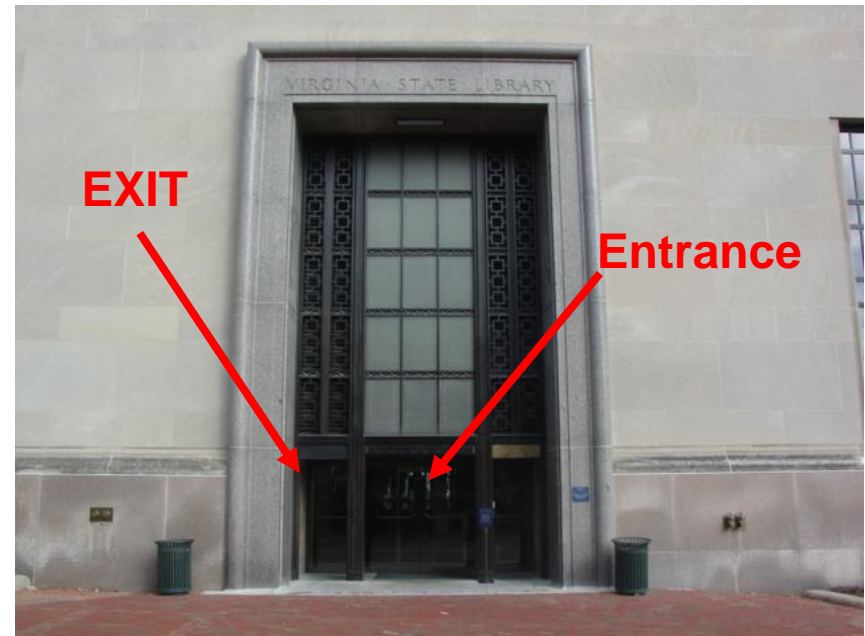
Darden Garden Doors (South side of the PHB)
